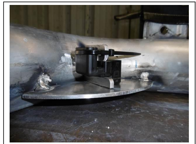
Figure 8: Fit sensors into protection bar.
